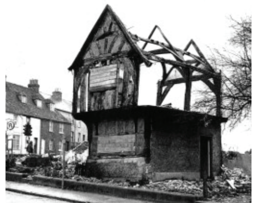
Demolition of Number 88 Milford Street to make way for the Milford Street Bridge and Ring Road
